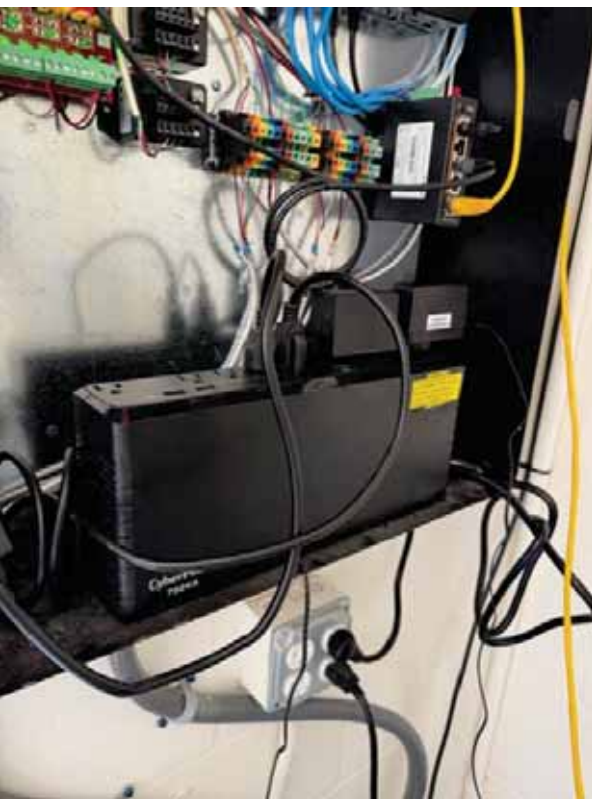
Battery Backup Replaced.
