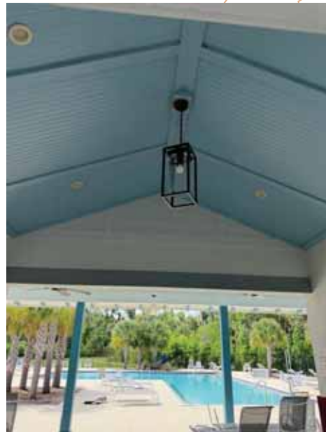
Pool Entrance Light Installed.
