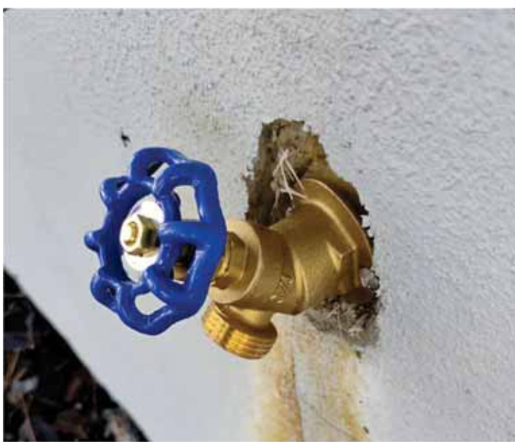
Hose Bib Replacement
