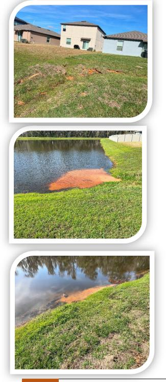
The area around the pond close to Yellow Trail has washed out again after being repaired.
