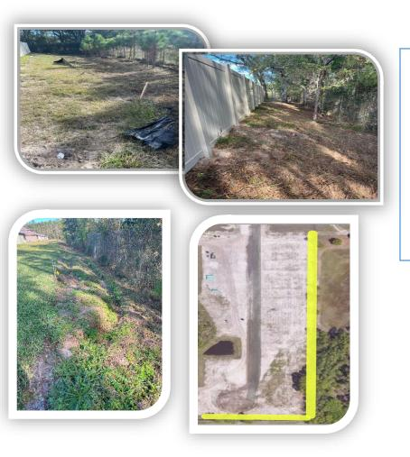
The area between the homeowner's property and the fence has not been graded, and no sod has been laid for maintenance.
